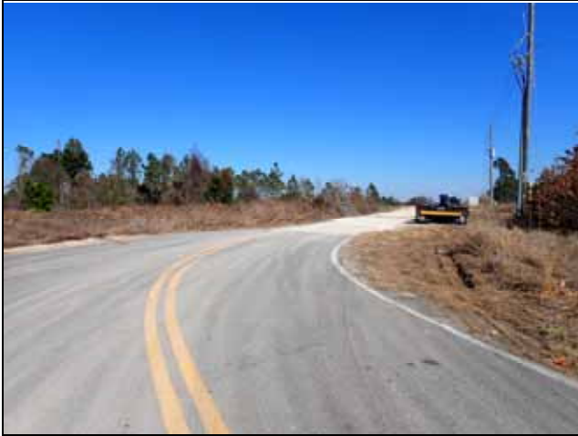
Paved Portion of Turkey Farm Rd.
