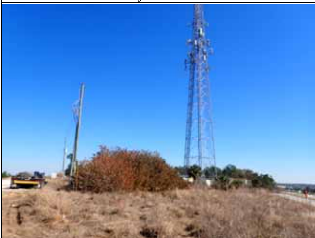
Communication Town Bisecting Subject Property
