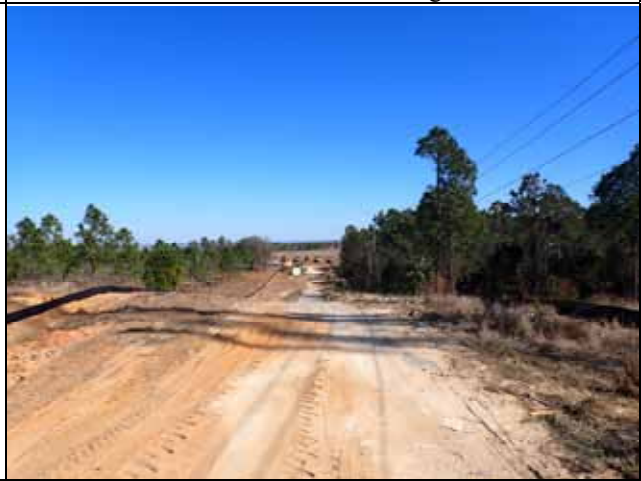
Unpaved Portion of Turkey Farm Rd.
