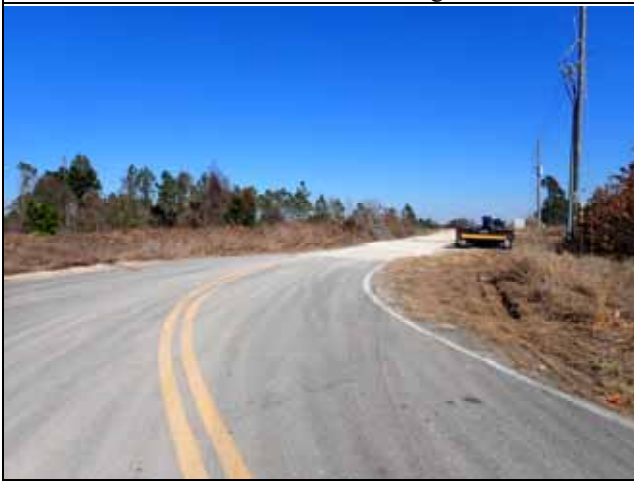
Paved Portion of Turkey Farm Rd.
